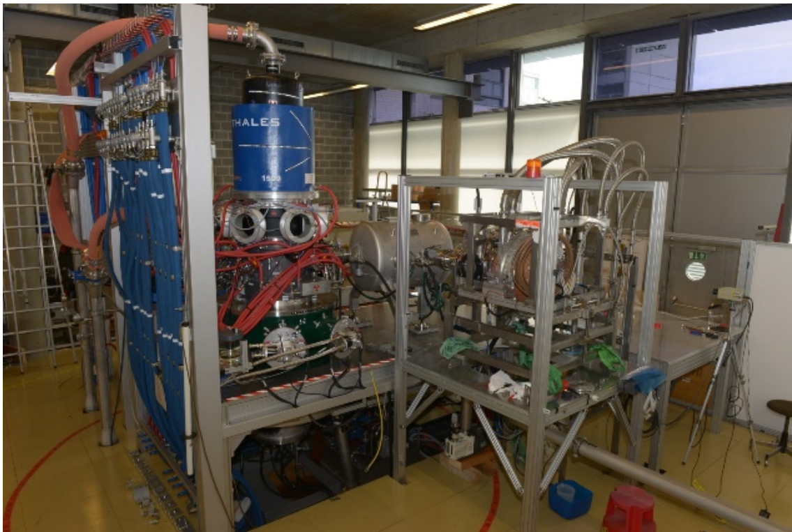
Figure 14: The prototype 1MW European gyrotron installed undergonig test in the new "Falcon" facility at the Swiss Plasma Center in Switzerland
